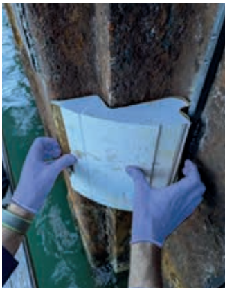
Application of Foam Filler.
