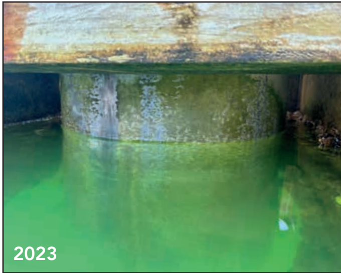
View of the SeaShield protected pile from underneath the floating wharf.
