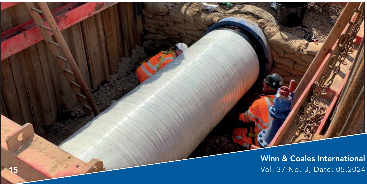
Below: Completed application of Denso Glass Outerwrap.
