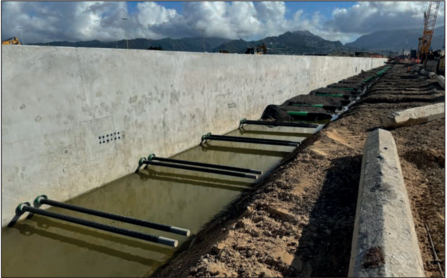
Above: The Denso™ wrapped tie rods are first installed and then...Below: Protected with PVC piping before final burial.
