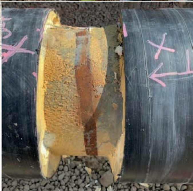
The field weld area before surface preparation.
