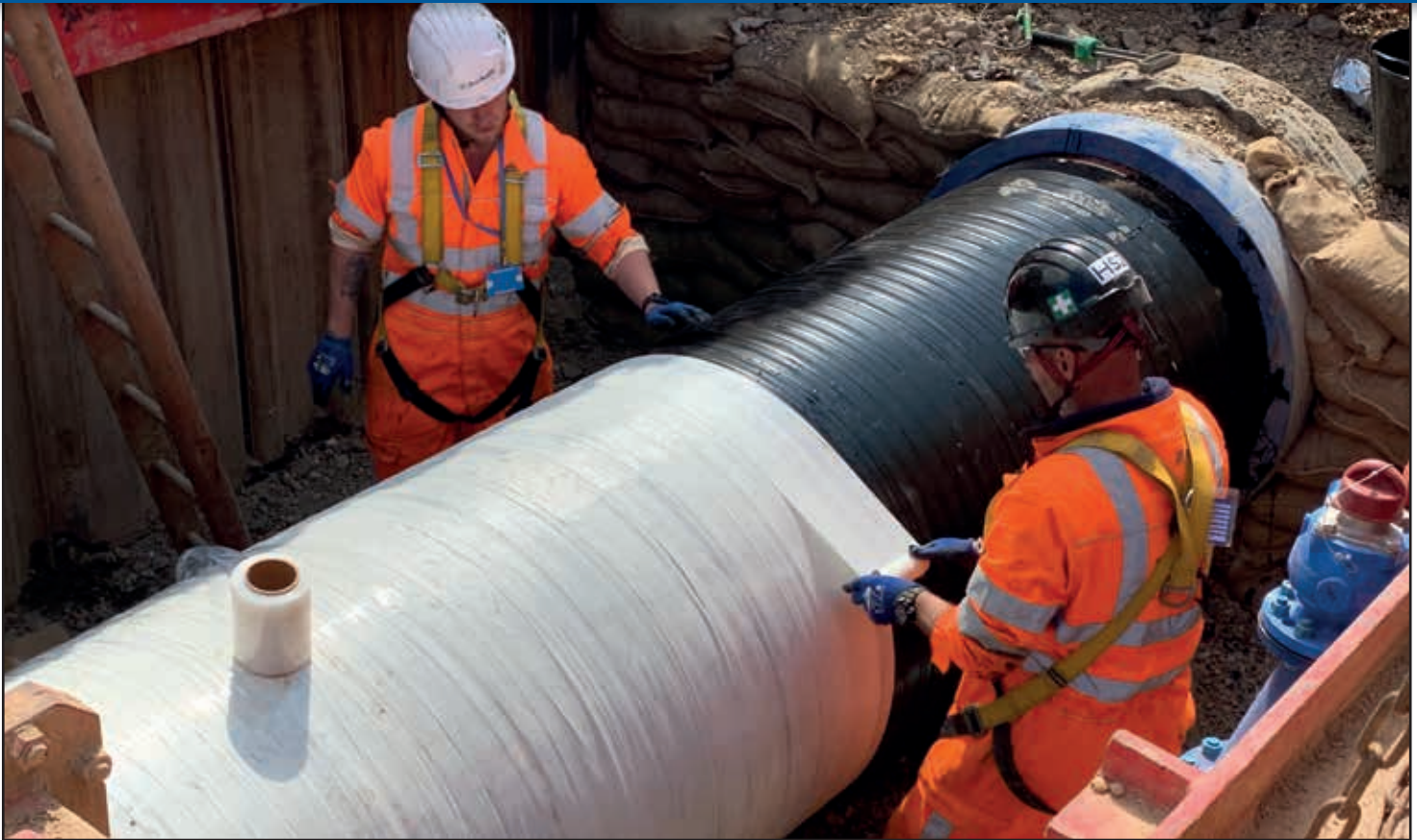
Above: Denso GOW is applied in a similar fashion, with a double layer of Denso Clear Outerwrap applied to aid curing and later removed.
