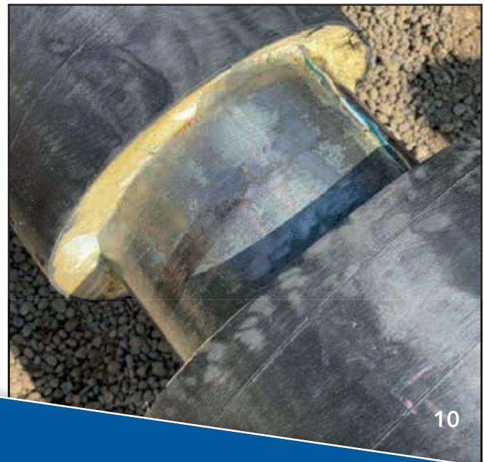
The field weld area after surface preparation.
