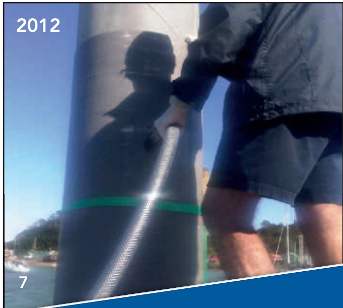
Below: Pumping the SeaShield Epoxy Grout into the 12.5mm annulus...
