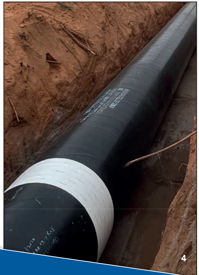
Below: Completed field joint wrapped with our Denso™ Liquid Field Joint Coating System.
