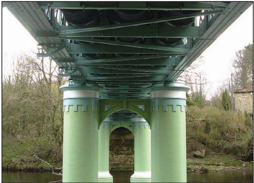
Above and below the Denso Steelcoat System protected aqueduct, matching the original colours as specified by the local authority to comply with the listed structure regulations.
