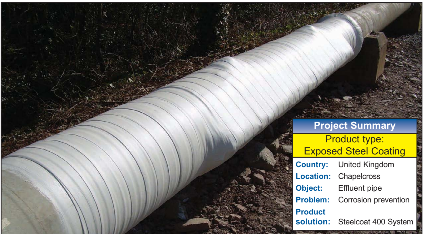
Below: The completed Steelcoat 400 System.
