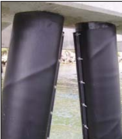
Pile protected with Denso's SeaShield Series 2000HD.
