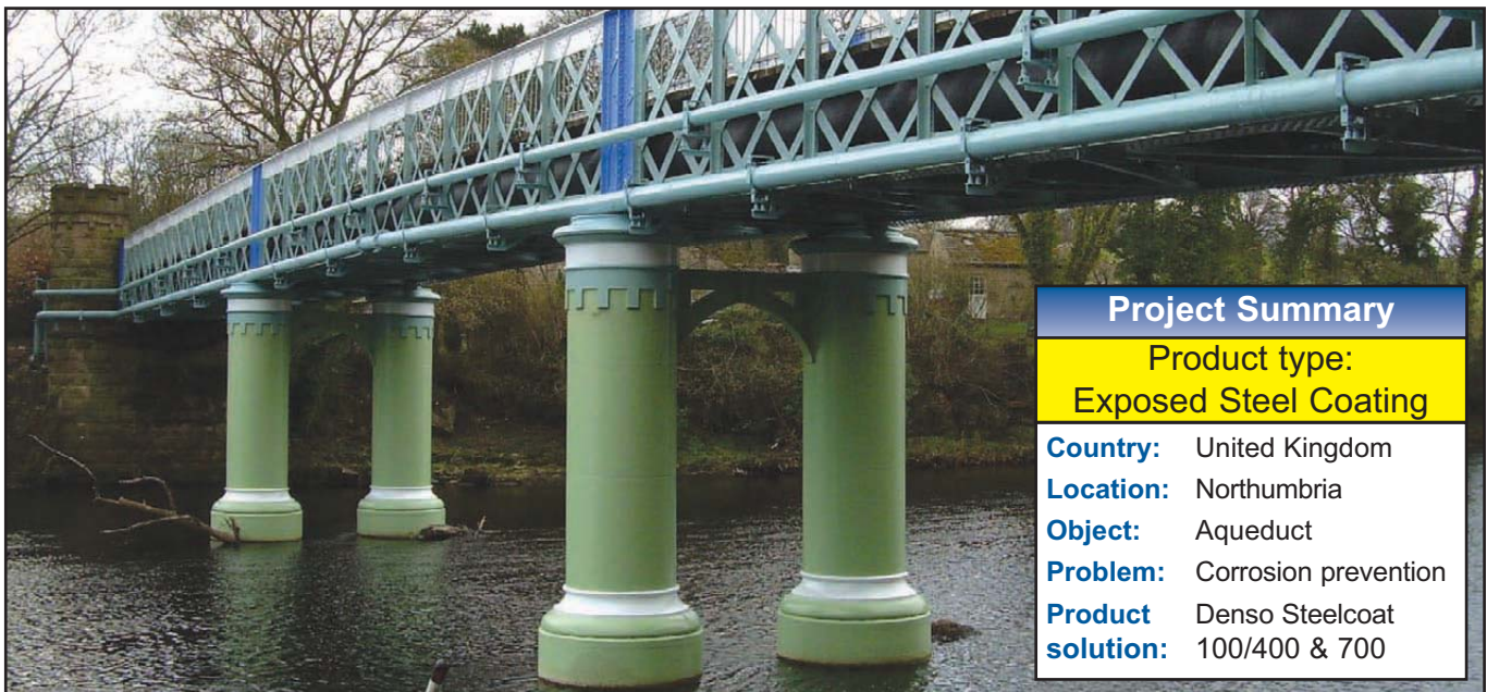
Above and below the Denso Steelcoat System protected aqueduct, matching the original colours as specified by the local authority to comply with the listed structure regulations.
