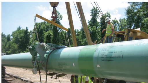
Automatic Spray Ring moving to the next joint.
