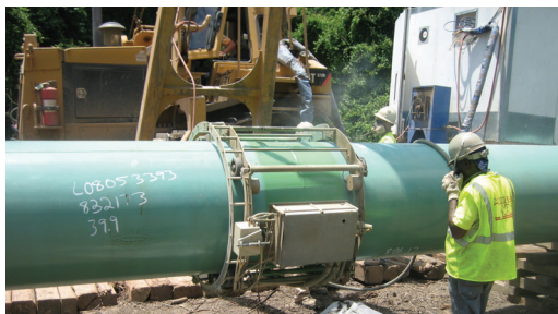
Spray applying Protal™ 7200 to 36" girth weld in 35 seconds.
