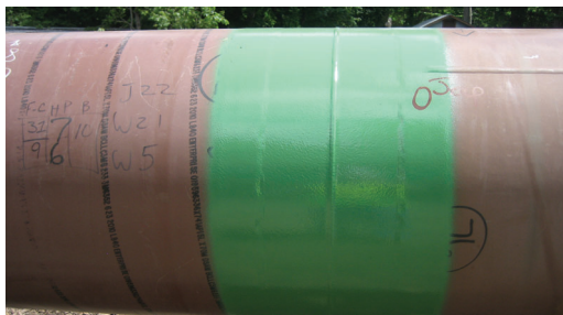
Protal™ 7200 applied at 24 to 32 mils DFT.
