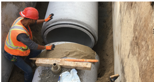
Denso LT Tape will remain flexible and continue to seal, even if the concrete cracks.
