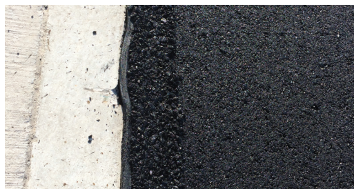
DensoBand™ provides a uniform, watertight, flexible seal.
