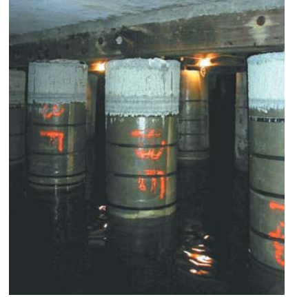
Structurally repaired timber piles with rebar, concrete and translucent SeaShield Fiber-Form fiberglass pile jackets.
