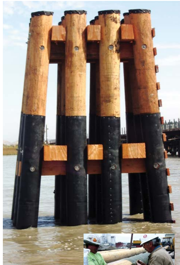
SeaShield Series 90 consists of Denso Marine Piling Tape preventing marine borer destruction and an outcover for mechanical protection of tape.
