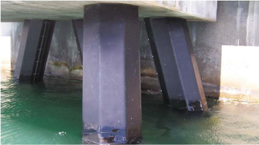
SeaShield Series 2000HD System was used to protect octagonal concrete bridge piles.
