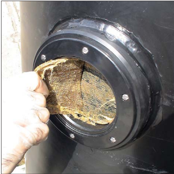
With the cover removed the petrolatum tape layer can be cut back to expose the pile surface for inspection.
