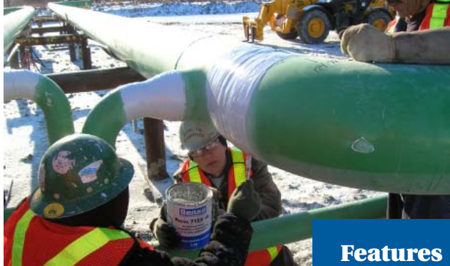
Protal 7125 being brush applied in arctic temperature conditions.
