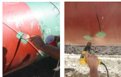
Protal Repair Cartridge application.
