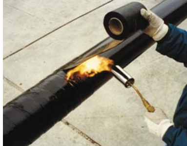
Pipeline rehabilitation and repair.
