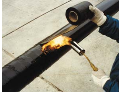
Pipeline rehabilitation and repair.
