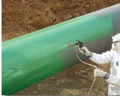
High build (up to 70 mils in one coat).
