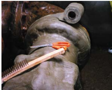
Applied to marginally prepared surfaces (SSPC SP2-3).
