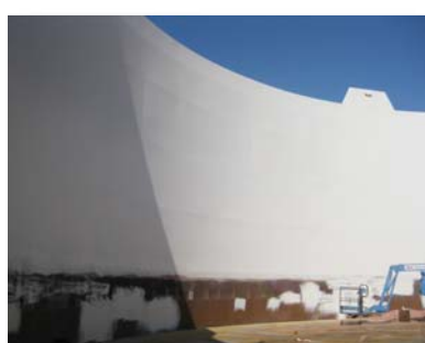
High build up to 40 mils in one coat.
