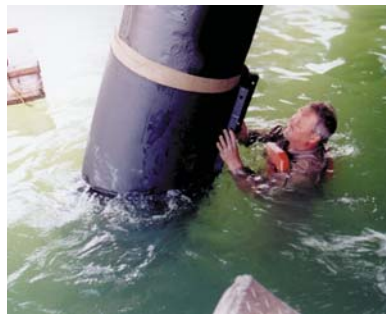
Low cost rehabilitation.
