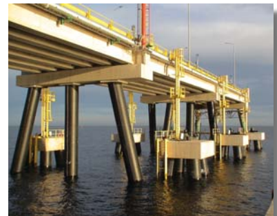
Adds years of life to pier and bridge structures.
