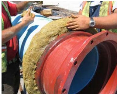
Minimal surface preparation (SSPC SP 2-3).
