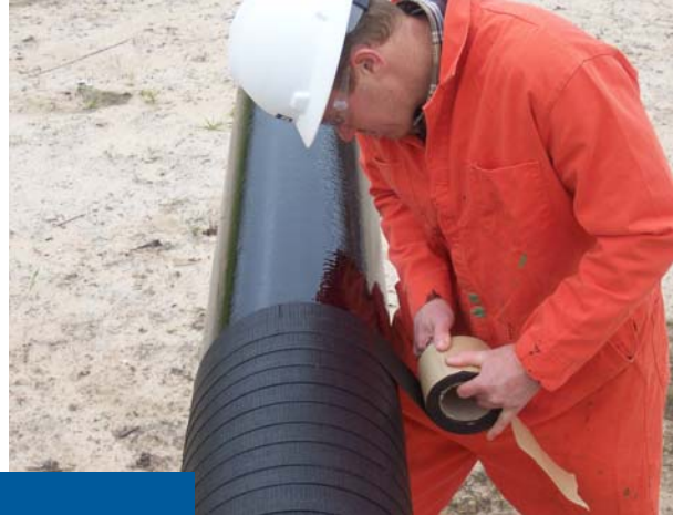
Application of Denso MB-50 Tape.
