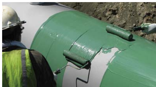
Applied with low nap rollers, to an average thickness of 30-35 mils.
