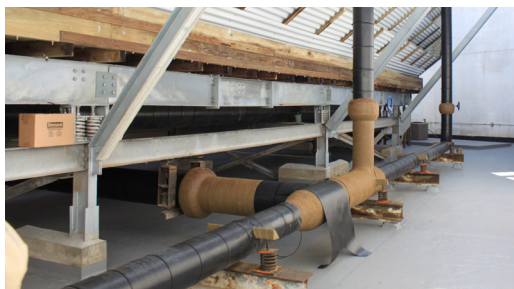
Overview of the complete Denso corrosion protection system for cooling towers for pipes, valves and fittings.
