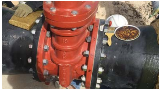
Surface prepared in accordance to SSPC SP-2/ SSPC SP-3 prior to application of the Denso Paste.
