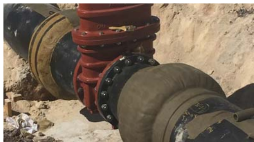
Application of the Densyl Tape over Profiling Mastic on the flanges.
