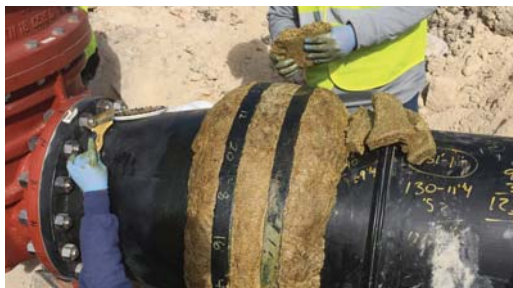
Application of the Denso Profiling Mastic creating a smooth profile for the Densyl Tape.
