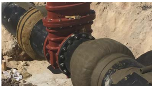
Application of the Densyl Tape over Profiling Mastic on the flanges.
