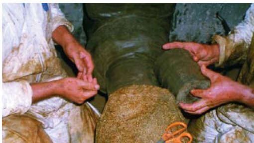
Densyl Tape is applied over the smooth contours of the Denso Profiling Mastic.
