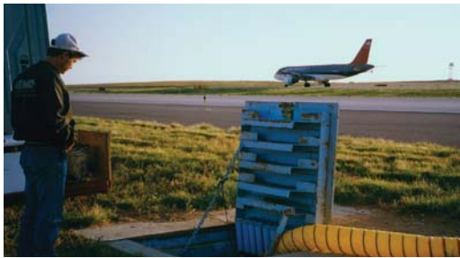
One of the 204 vaults in close proximity to the airport runway.
