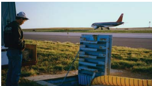
One of the 204 vaults in close proximity to the airport runway.
