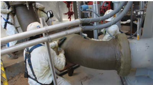
Denso Paste S105, Profiling Mastic and Densyl Tape applied to all flanges and valves.
