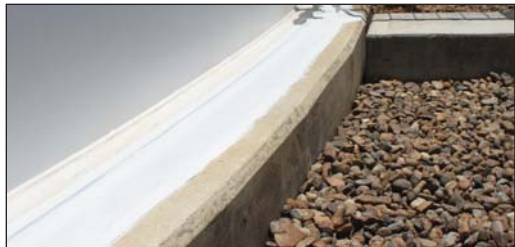
Finished tank with Denso Weathershield 55 applied as a top coat completing the system.
