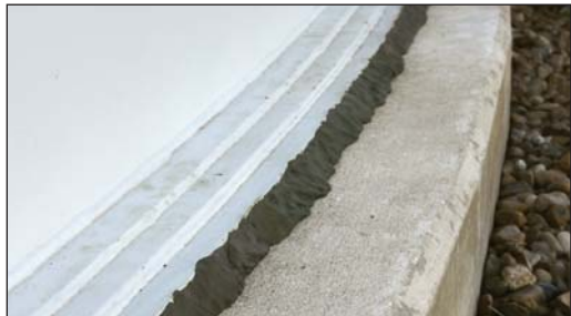
Tank plinth area seal with Densyl Mastic to prevent moisture from entering.
