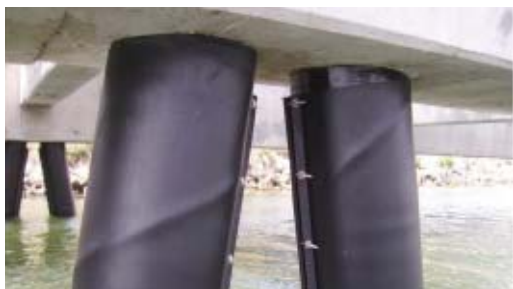
Pile protected from with Denso's SeaShield Series 2000HD.
