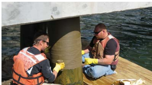
Wrapping the prepared pile with Denso Marine Piling Tape.
