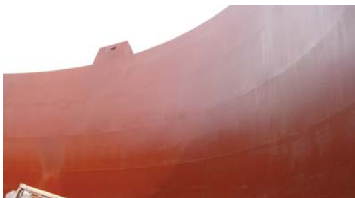
Open top tank, side walls primed with 400.
