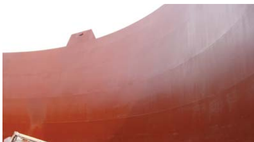
Open top tank, side walls primed with 400.
