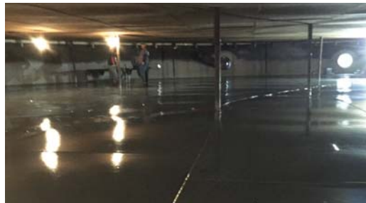
Archco 476 is high temperature internal epoxy phenolic-novolac lining for tanks and pipes.
