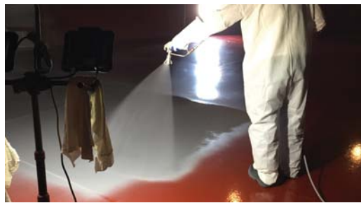
Archco 476 being sprayed applied over Archco 400.
