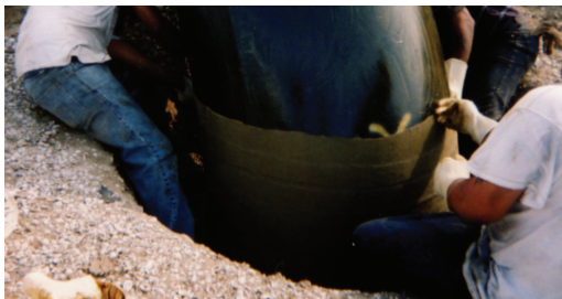
Densyl Tapes provides long term corrosion protection to pipes, flanges, valves and related surfaces.
