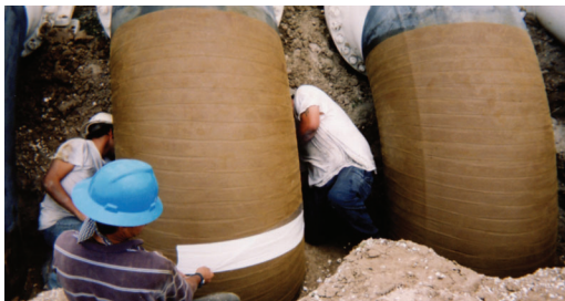
Densyl Tape and Denso Glass Outerwrap is easily applied by hand and requires no special training or equipment.
