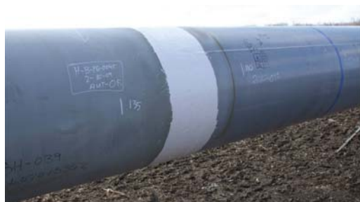
Coated girth weld with Protal 7125.
