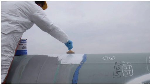
Applying Protal™ 7125 by brush.
