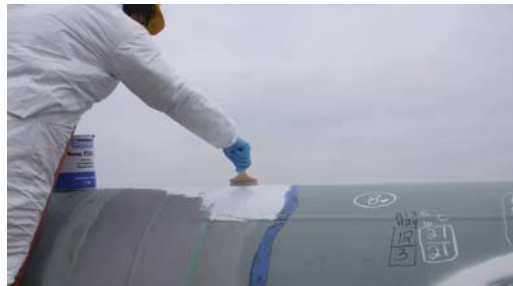
Applying Protal 7125 by brush.
