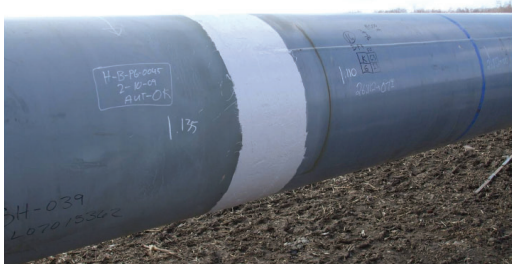
Coated girth weld with Protal™ 7125.
