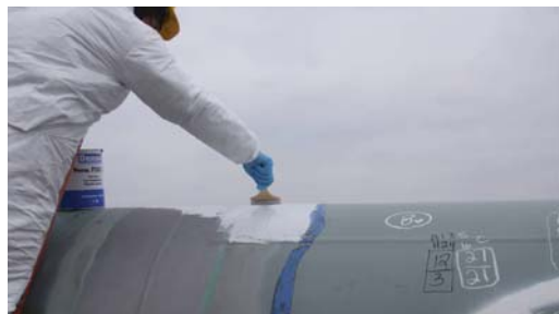
Applying Protal 7125 by brush.
