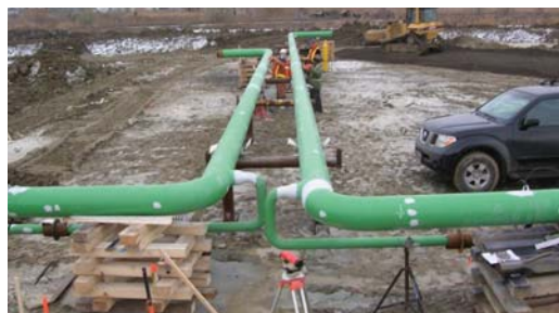
Holidays FBE pipe repaired with Protal 7125.
