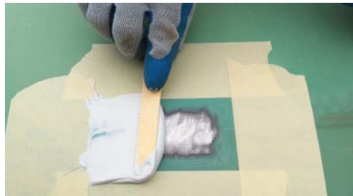
Application of Protal 7125 for holiday repair of FBE.
