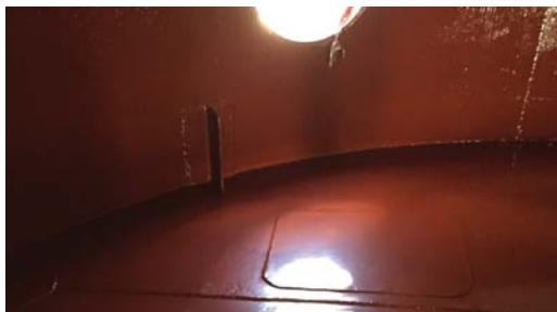
Archco 400 Primer applied to tank substrate.
