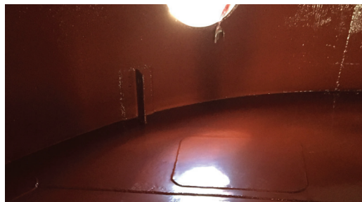
Archco™ 400 Primer applied to tank substrate.
