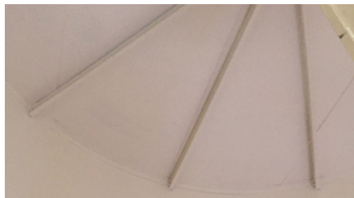
Archco™ 453HT applied to the tank roof at 30 mils DFT average.
