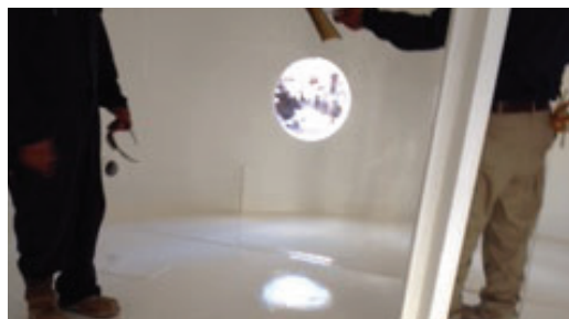
Holiday testing the Archco™ 453HT coating and confirming it was pin-hole free.
