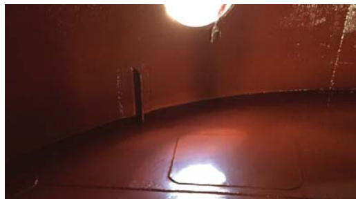
Archco 400 Primer applied to tank substrate.
