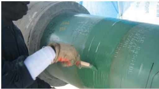
Protal 7200 brush applied to 30 mils at 180°F.
