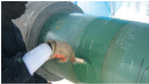
Protal™ 7200 brush applied to 30 mils at 180°F.
