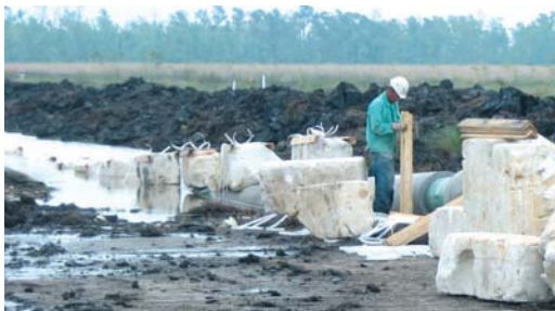
Protal 7200 is cured and holiday detected within 15 minutes.
