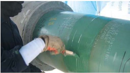
Protal 7200 brush applied to 30 mils at 180°F.
