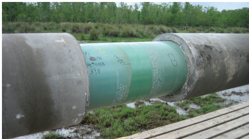
Pipe is pushed into the water 20 to 30 minutes after coating application.
