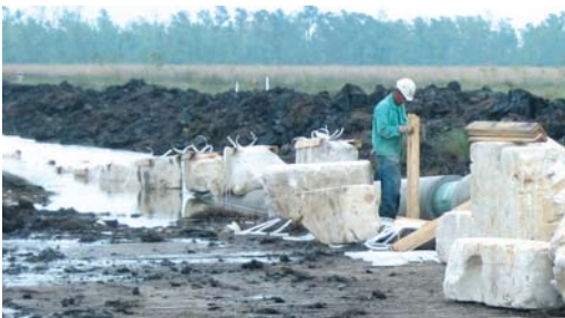
Protal 7200 is cured and holiday detected within 15 minutes.
