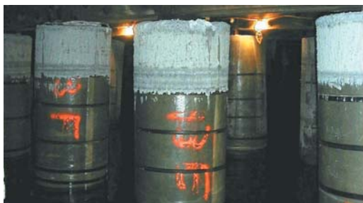
Completed SeaShield Fiber-Form system.
