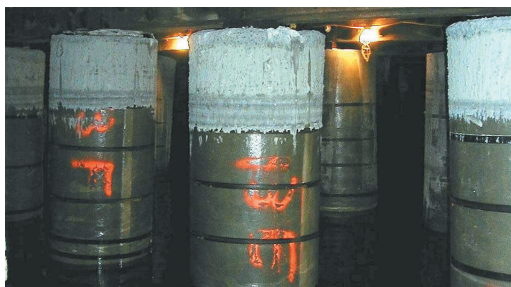
Completed SeaShield™ Fiber-Form system.
