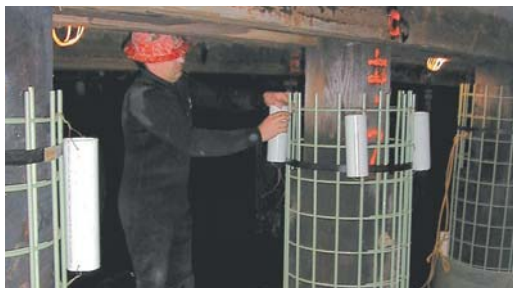
The SeaShield Fiber Forms are positioned around the timber piles.
