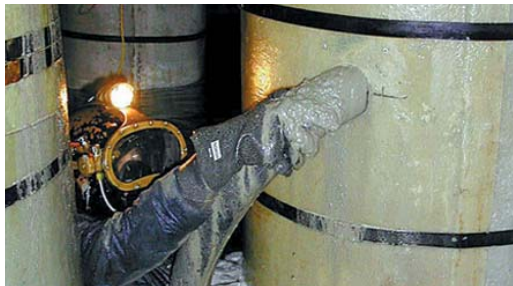
Concrete is pumped into the annulus space between the jacket and timber pile.
