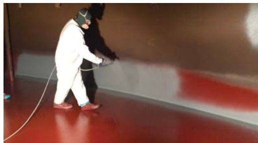
Archco 476P sprayed applied over the primer to provide chemical and high temperature resistances.
