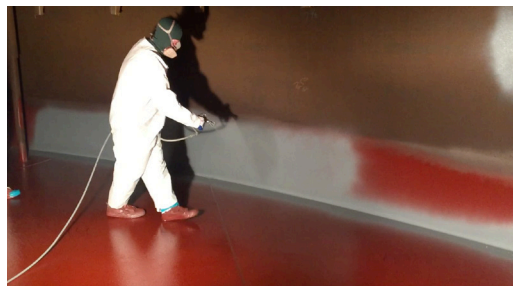
Archco 476P sprayed applied over the primer to provide chemical and high temperature resistances.
