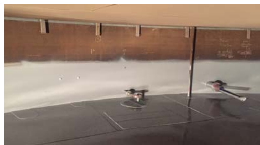
Fully cured Archco 476P lining allowing the tank to return to service within 8 hours.
