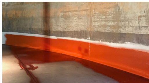
Archco 400 primer being applied to the blasted floor and side walls of the tank.
