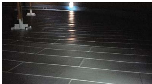
Pipeline storage company, 220' fuel oil tank, outside Albany, New York, on the Hudson River.
