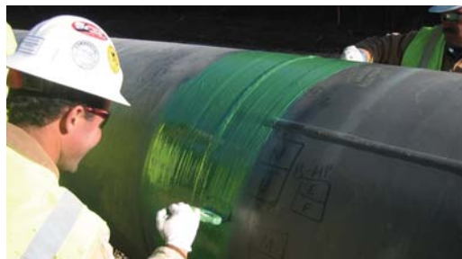
Brush applied coating protection of girth welds.
