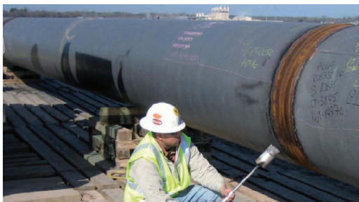
Pre heating of weld joints prior to blasting.
