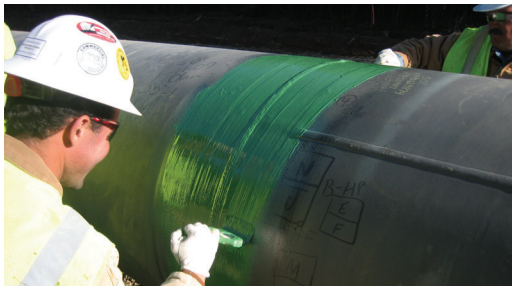
Brush applied coating protection of girth welds.
