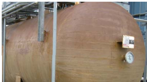
Denso Hi-Tack Tape and Primer applied to sweating ammonia tanks.
