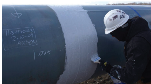
Applying Protal™ 7125 at 50 mils for directional drill on 42" diameter pipe.
