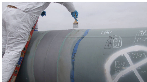
Applying Protal™ 7125 by brush.
