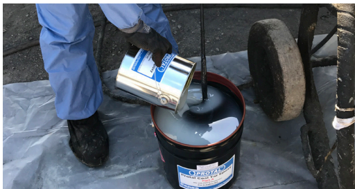
Protal 600 CTE Part "A" & "B" being mixed prior to the spray application.
