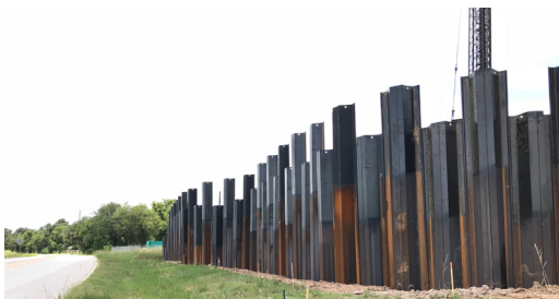
Sheet Piles coated with Protal 600 CTE being driven into place.
