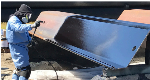
Application of Protal 600 CTE using a single leg airless spray pump.
