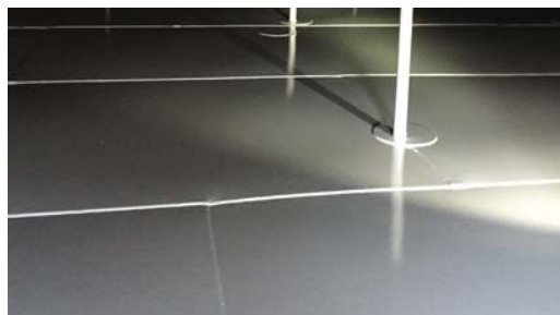
Finished Archco 400/400HB tank lining.
