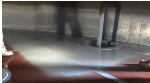
Spraying Archco 400HB over the 400 primer.
