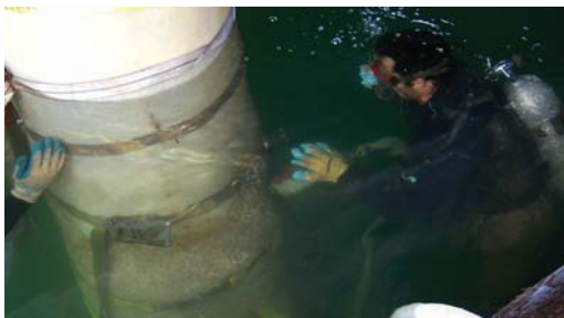
Pumping 550 Epoxy Grout.
