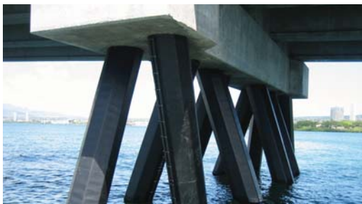
Series 2000HD protecting octagonal piles.
