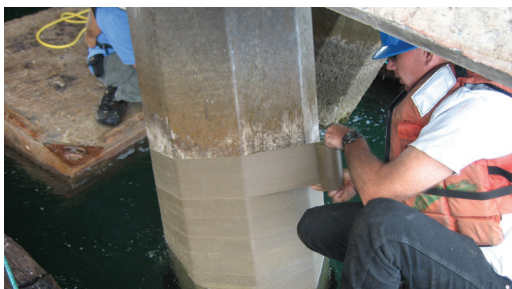
Denso Marine Tape applied before application of Series 2000HD outercover.
