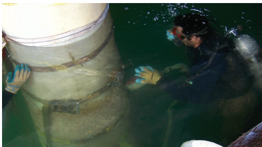
Pumping 550 Epoxy Grout.
