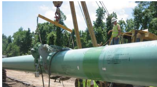
Automatic Spray Ring moving to the next joint.
