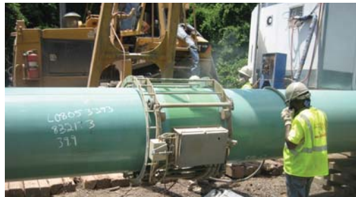
Spray applying Protal 7200 to 36" girth weld in 35 seconds.
