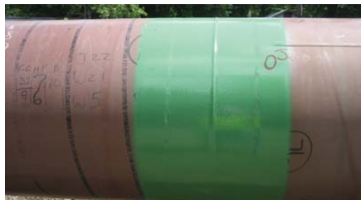
Protal 7200 applied at 24 to 32 mils DFT.
