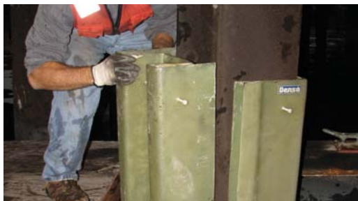
Installation of the two Fiber-Form half shells around a steel h-pile.
