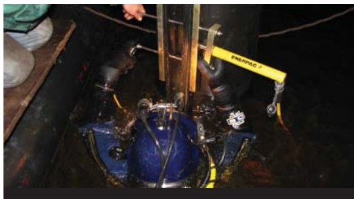
Installation of HDPE jacket and hydraulic tensioning system.
