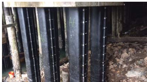
Completed H-Piles fully protected with the SeaShield Series 2000HD System.
