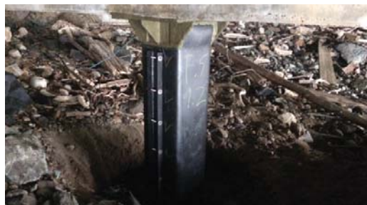
Pile cap/gusset area protected with the SeaShield SplashZone UW Epoxy.
