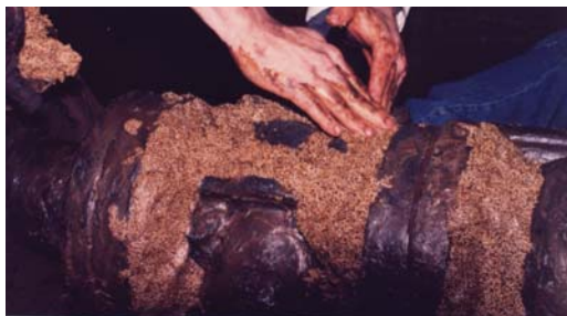
Denso Profiling Mastic easily conforms around irregular shapes and covers sharp edges.
