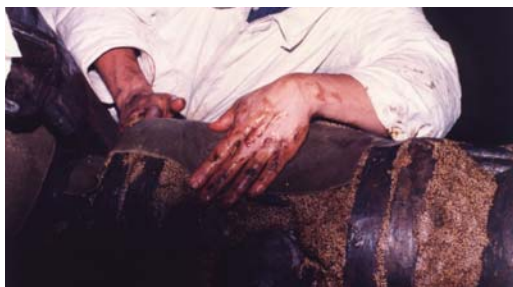
Over 100 water valve assemblies were protected with Denso Petrolatum Tape System.
