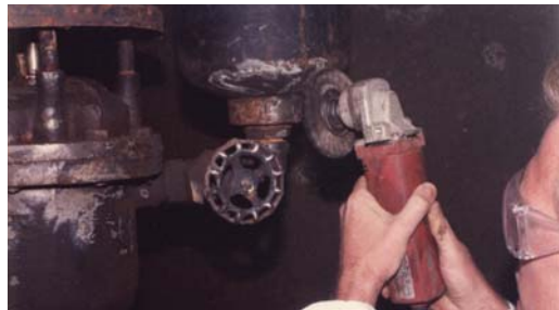
Valves and fittings are cleaned by hand tool cleaning.
