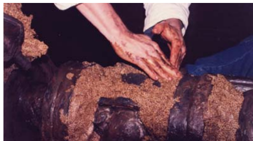
Denso Profiling Mastic is applied to provide a smooth profile.
