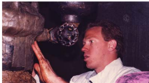
Over 100 valves and fittings were protected with the Denso Petrolatum Tape System.
