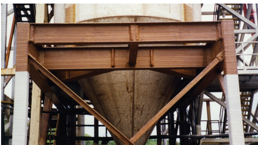
Denso Petrolatum Tape products fully protecting over 10,000 sq. ft. of steel head frame.
