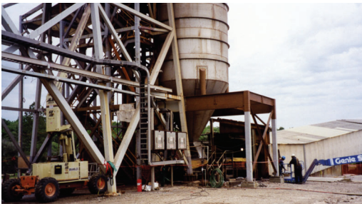
The Cargill Salt Head Frame which has been in operation since 1954.
