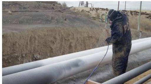
Archco 453HT being sprayed applied out in the field.
