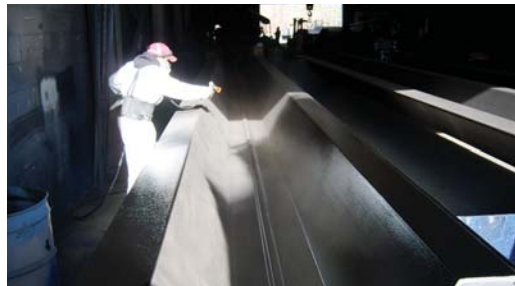
Spraying Denso Rigspray to sheet pile.
