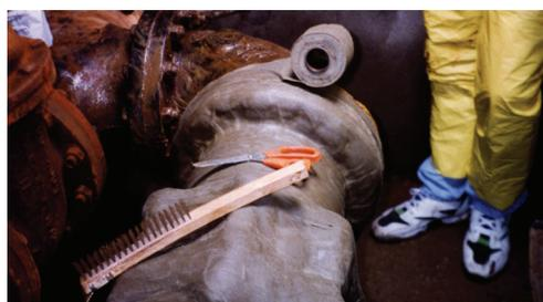
All surfaces were prepared by hand tool cleaning.
