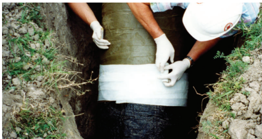
Denso Glass Outerwrap is easily applied by hand and requires no special training or equipment.
