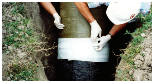
Denso Glass Outerwrap is easily applied by hand and requires no special training or equipment.
