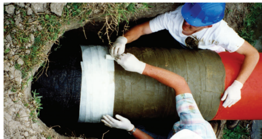
Denso Glass Outerwrap, which is resistant to water, acid, salts and soil organics.
