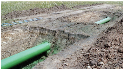
Spray applied Protal™ 7200 protects 600 liner feet of 36" diameter pipe.
