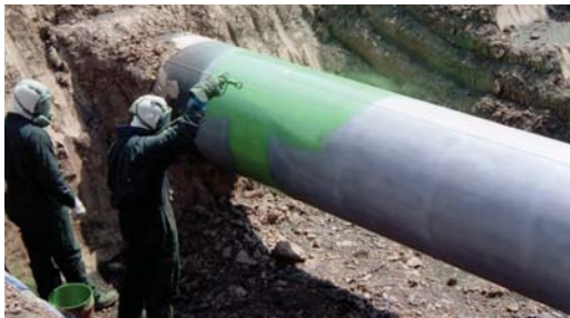
Protal 7200 being sprayed applied in the field.
