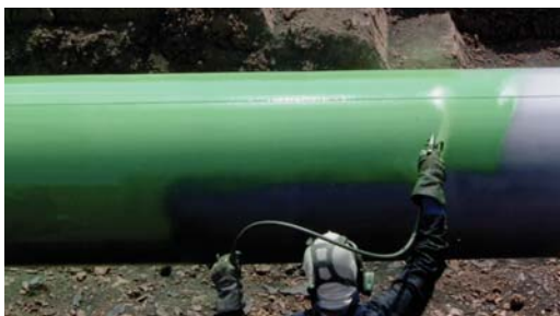
Protal 7200 is a high build (up to 50 mils) liquid epoxy coating.
