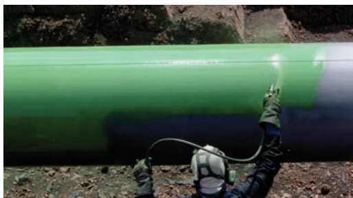
Protal 7200 is a high build (up to 50 mils) liquid epoxy coating.
