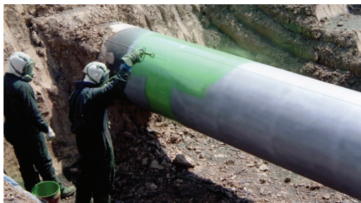
Protal™ 7200 being sprayed applied in the field.
