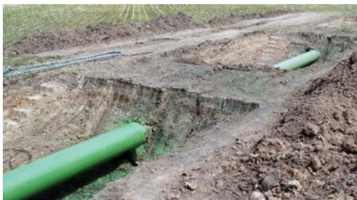
Spray applied Protal 7200 protects 600 liner feet of 36" diameter pipe.
