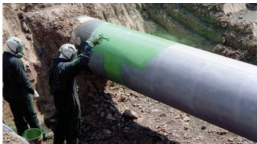
Protal 7200 being sprayed applied in the field.
