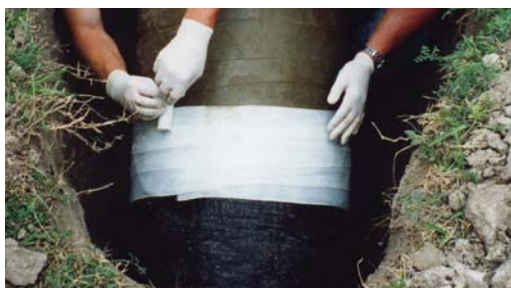
Denso Glass Outerwrap applied spirally over the Densyl Tape.
