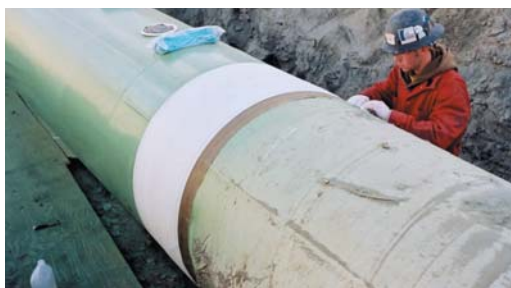
Used as a tie-in or interface coating between dissimilar coatings.
