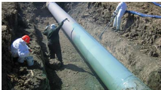
Pipe being spray applied with Protal 7200.
