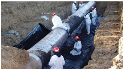
Removal of old coal tar enamel coating.
