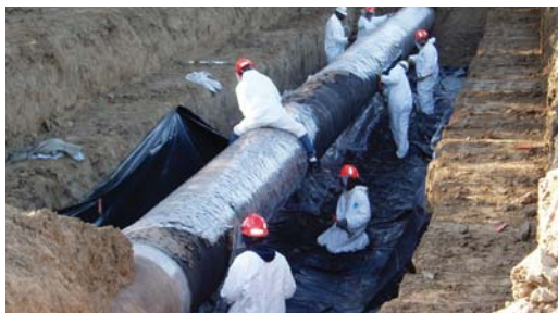
Removal of old coal tar enamel coating.
