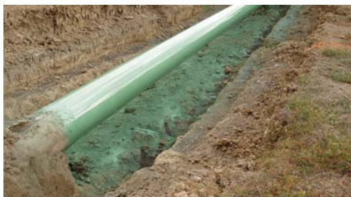
Section of pipe with newly coated Protal 7200.
