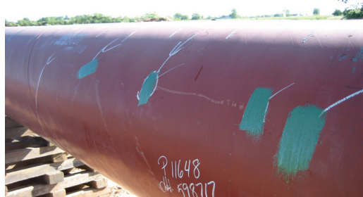
Repairing “holidays” with Protal™ 7200 Repair Cartridge.
