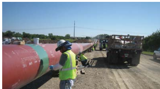
Mainline crew applying Protal 7200 to girth welds.
