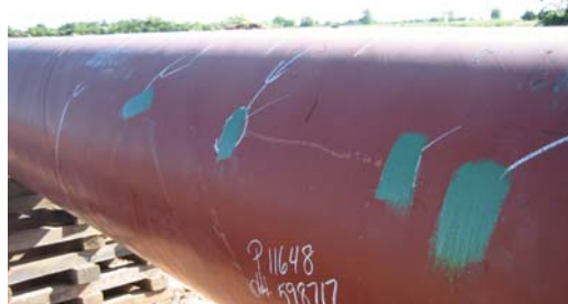
Repairing "holidays" with Protal 7200 Repair Cartridge.
